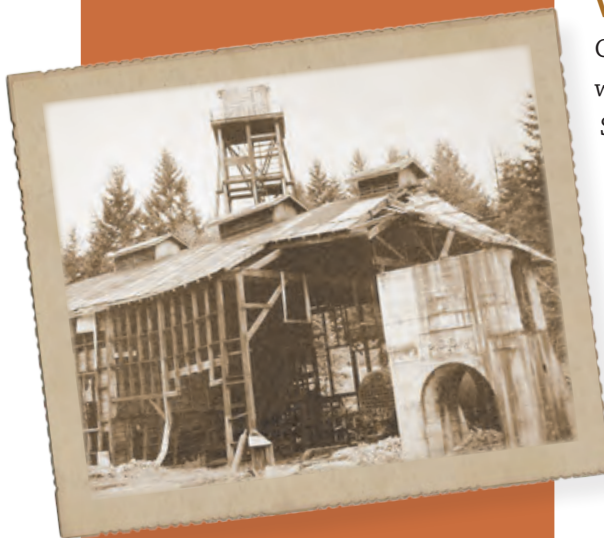
Morden circa 1950-60, Boiler House remains, Water Tower.
